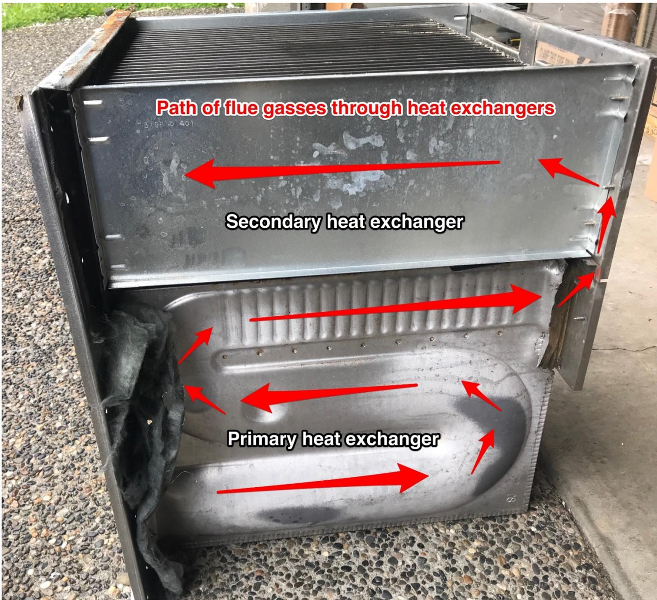
**Image 3** – Removed heat exchanger assembly (upside down from installed orientation) showing the path the flue gasses travel through the heat exchangers.
